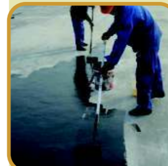
Substrate treatment: Brush the coatings directly after cleaning up the substrate normally. If necessary, brush the specialized primer on the substrate.
