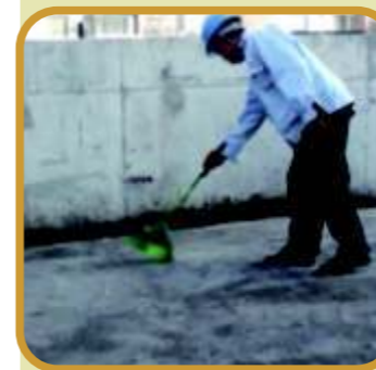
Substrate cleaning: Cleaning up the sundries and dust.
